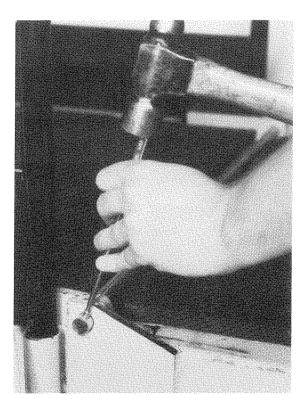
Figure 13. Expanpin Installation.
